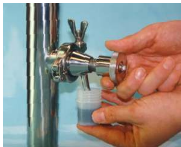
Sampling from a downpipe
